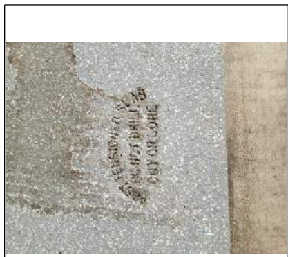
Post-tensioned concrete stamp (GARAGE floor)
