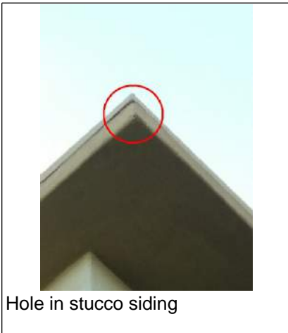
Hole in stucco siding
