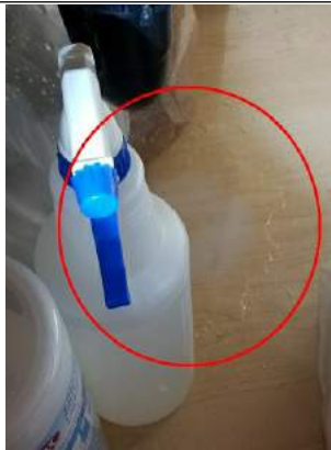
1st Floor, RIGHT FRONT Bathroom (Active leak)
