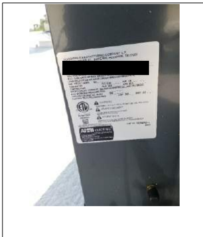
Electrical conduit separated from unit
